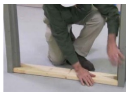
FIG. 11 – TEMPORARILY BRACE FRAME
