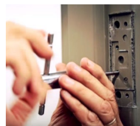
FIG. 27 – INSTALL IVES HINGE FIRST
