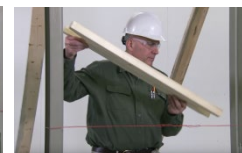
FIG. 13 – ADD MID-HEIGHT SPREADER
