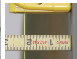
FIG 15. LAY BLOCK, CHECKING FOR PLUMB, LEVEL AND SQUARE EVERY TIME YOU MAKE AN ADJUSTMENT
