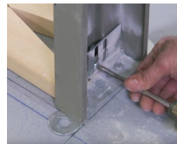
FIG. 11 – TEMPORARILY BRACE FRAME
