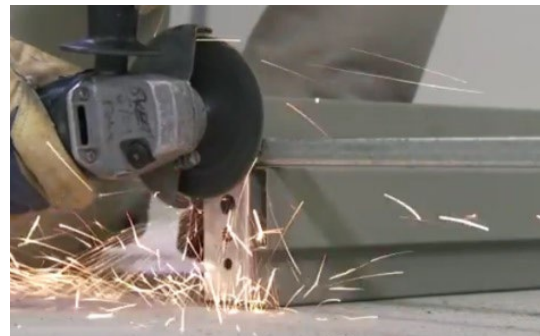
FIG. 8 – PROPERLY GRIND OFF SHIPPING BAR
