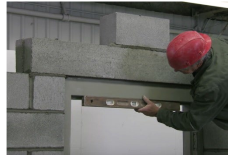
FIG. 19 – TYP A HIGH PSI PREFAB CONCRETE LINTEL IS USED, ALTHOUGH PROPER STEEL LINTELS MAY ALSO BE SPECIFIED. REF NON-TORNADO SDI/ALLEGION MASONRY INSTALL VIDEO min 7:50-8:30. ENSURE NO SAGGING.
